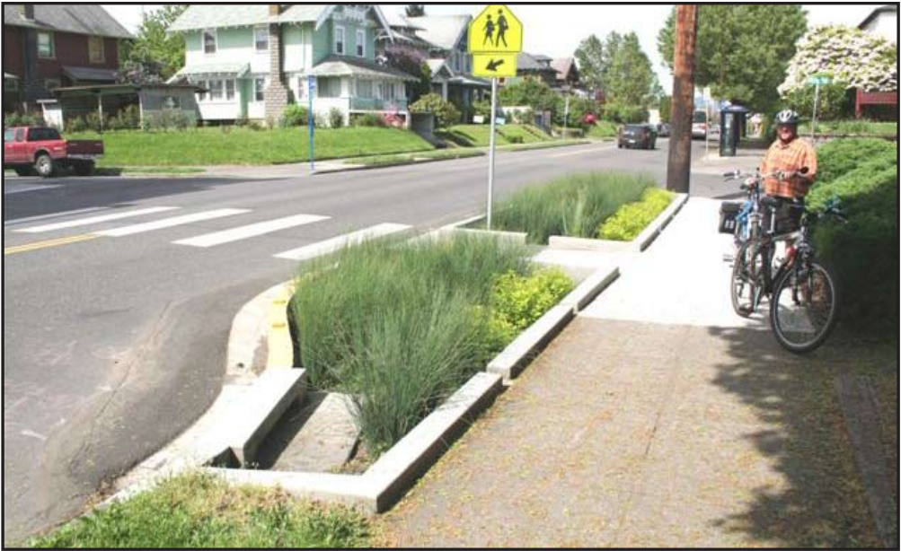
Roadside rain gardens are swale-like planted areas to mitigate stormwater runoff.
