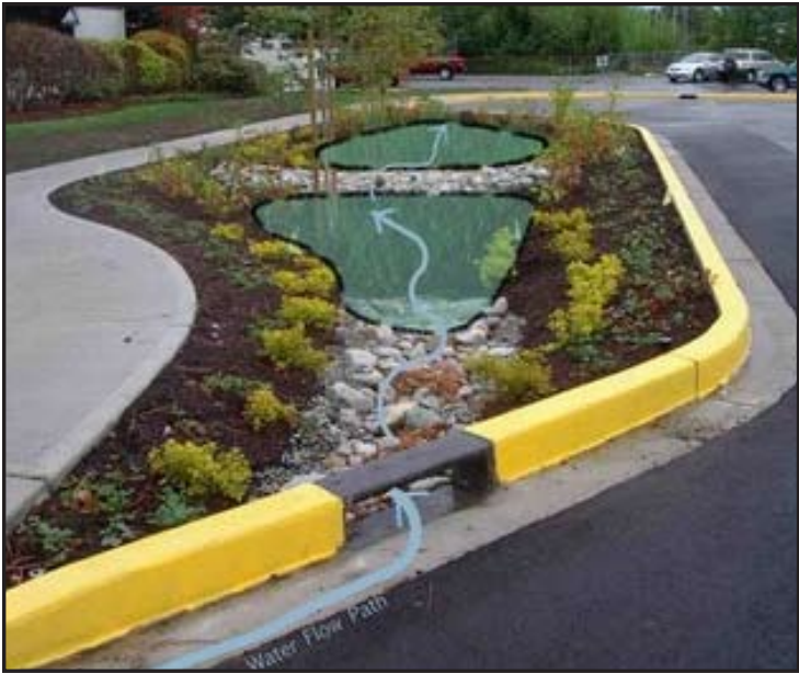
This bioswale area on the curb collects water in gravel/stone-filled channels on surface, filtering into the ground.
