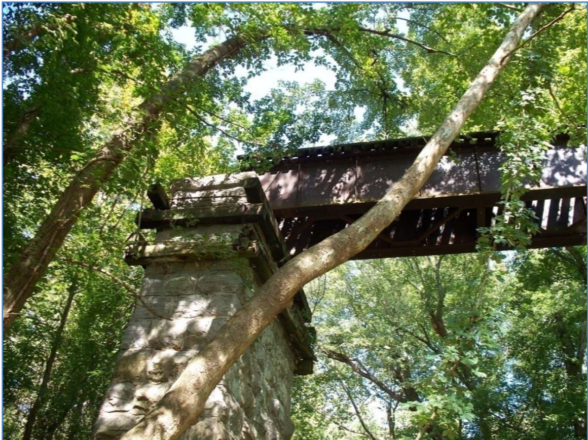
Figure 4-17 Remaining Structure over Brush Creek at MP 36.60
