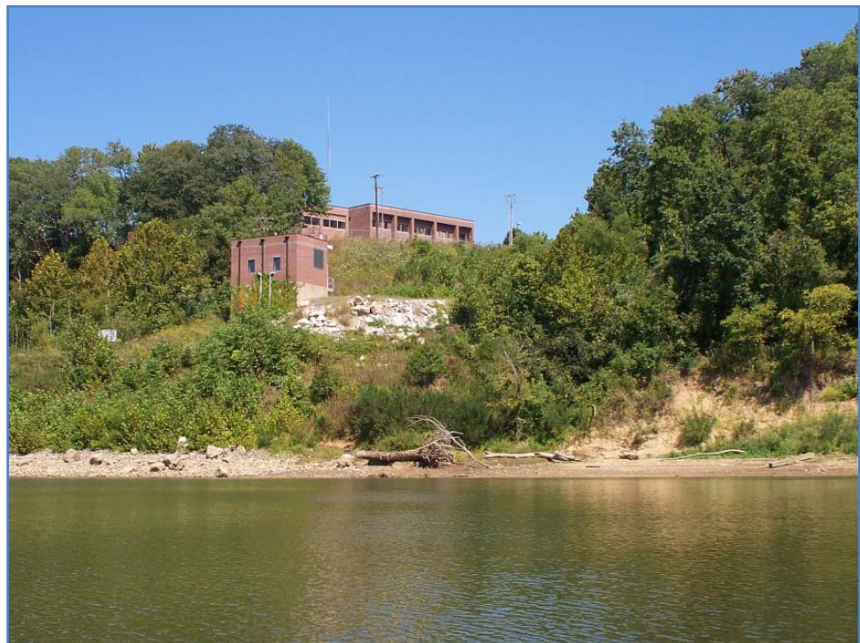
Figure 4-14 Clarksville Water Plant at MP 36.4
