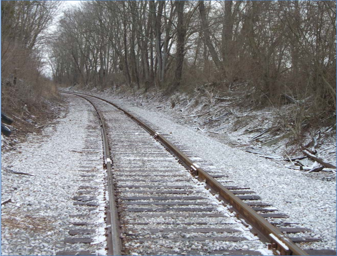
Figure 4-1 Nashville & Western Track near MP 7
