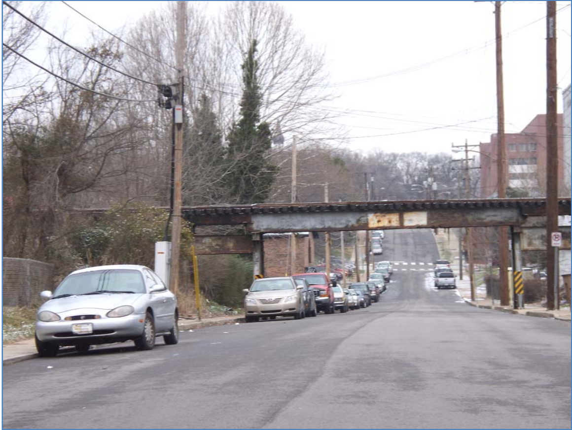
Figure 4-2 Meharry St. Bridge
