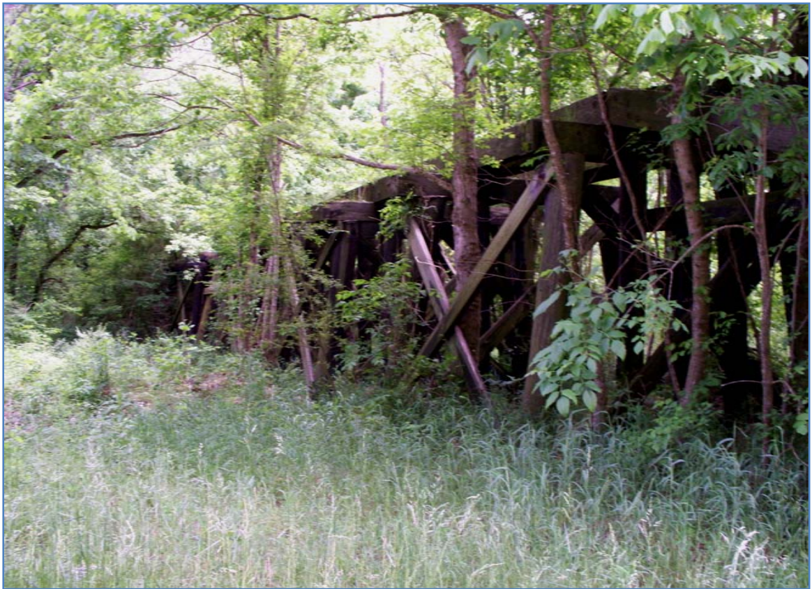
Figure 4-6- Chapmansboro Rd. Bridge at MP 21.97
