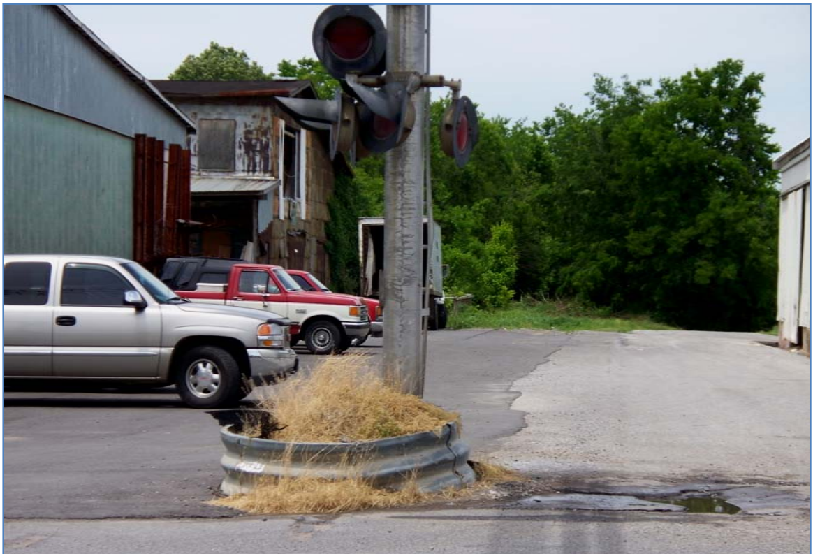
Figure 4-4 Track Adjacent to Hwy 49 in Ashland City
