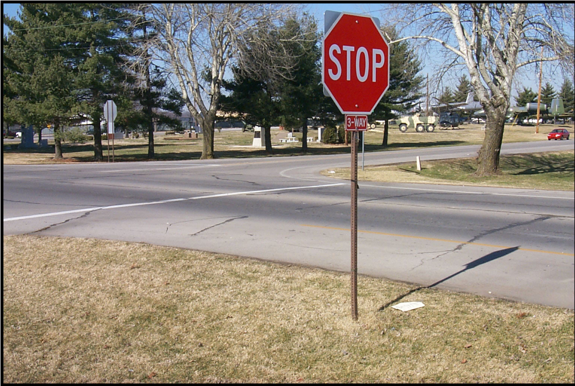
Exhibit 5.51 Normandy Boulevard and Kentucky Avenue. Note STOP sign is placed 33 feet in advance of Stopbar (northwestward view).
