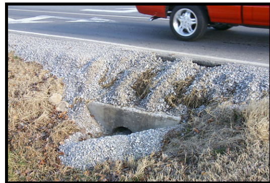
Exhibit 7.13 Example of undesirable drainage feature
