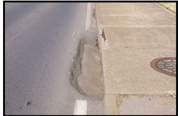
Exhibit 7.17 Example of undesirable drainage feature
