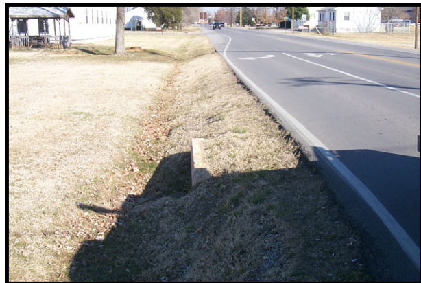
Exhibit 7.6 Example of severe side-slope
