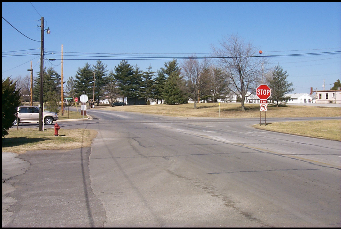
Exhibit 5.53 Screaming Eagle Boulevard and Tennessee Avenue. Note inappropriate use of “No Left-Turn” sign (northward view).
