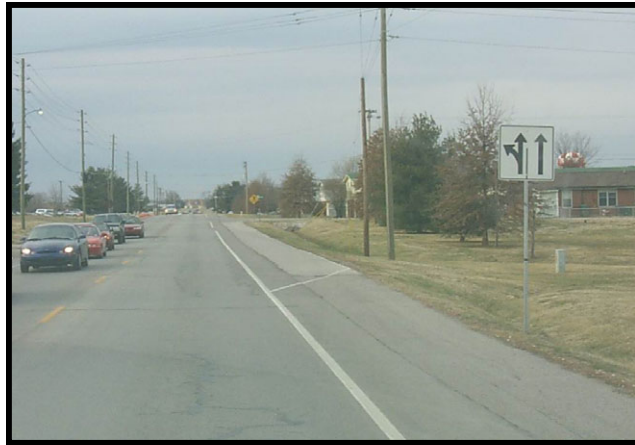
Exhibit 7.8 Example of inappropriate use of lane use control sign
