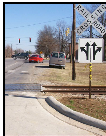
Exhibit 7.11 Example of two different types of messages on same signpost
