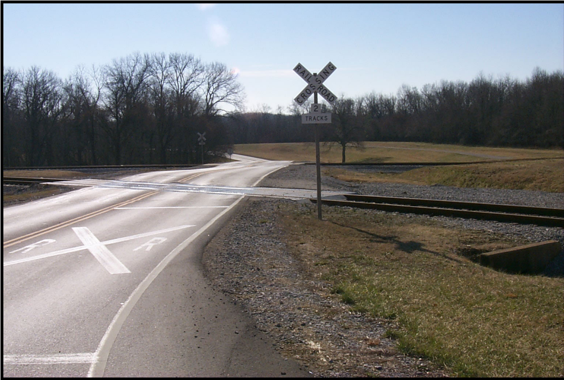
Exhibit 7.1 Typical grade crossing treatment, this from Wickham Avenue south of 1 st Street
