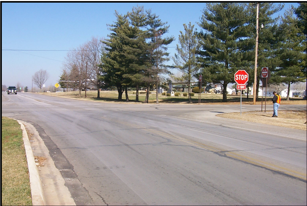
Exhibit 5.52 Normandy Boulevard and Tennessee Avenue. Note lack of One-Way signing for Normandy Boulevard (northward view).
