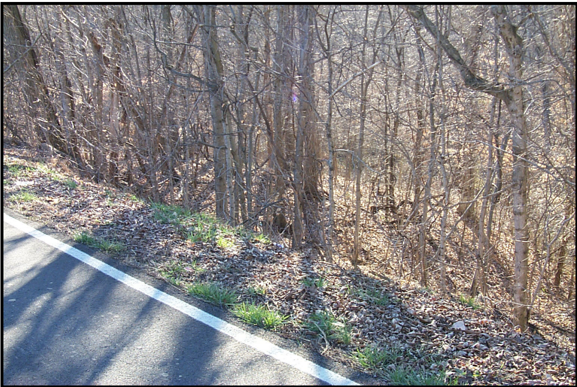
Exhibit 6.24 Unprotected dropoff along TN Route 233
