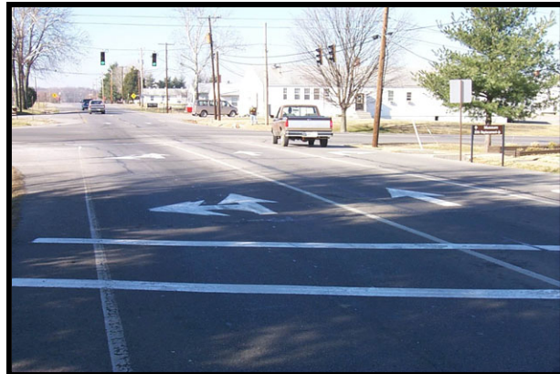
Exhibit 7.9 Example of white edge line on left side of traffic
