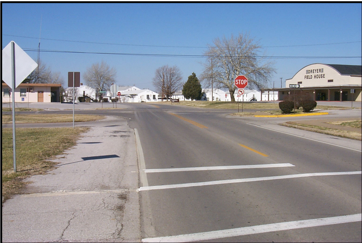
Exhibit 5.54 Screaming Eagle Boulevard and Kentucky Avenue. Note that crosswalk is not at intersection (northward view).
