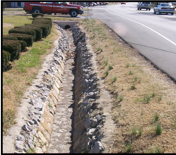
Exhibit 7.16 Example of undesirable drainage feature
