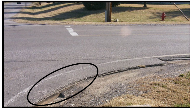
Exhibit 7.7 Example of edge drop-off (From intersection of Forrest Road and Reed Avenue)
