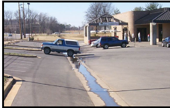
Exhibit 7.12 Example of undesirable drainage feature
