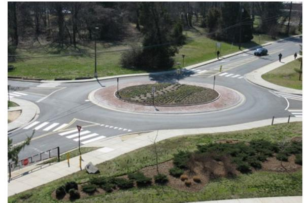
*Modern roundabout used to increase throughput (compared to signals) and lowers speeds overall. Photo source: Andrew Bossi*
