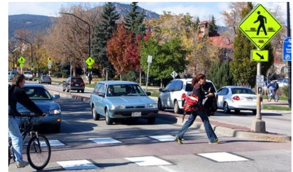
Flashing diodes in pavement\* and warning sign.
