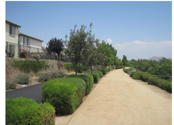
*This trail made of decomposed granite allows rainwater to flow through, preventing flooding, while providing a solid surface for walking and biking. Photo source: Mike Singleton*
