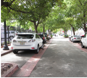
Valley gutters (red area). Credit: Ryan Snyder.
